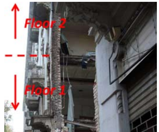
Façade of first floor thrust outwards – the area of maximum warping between the first and second floors
