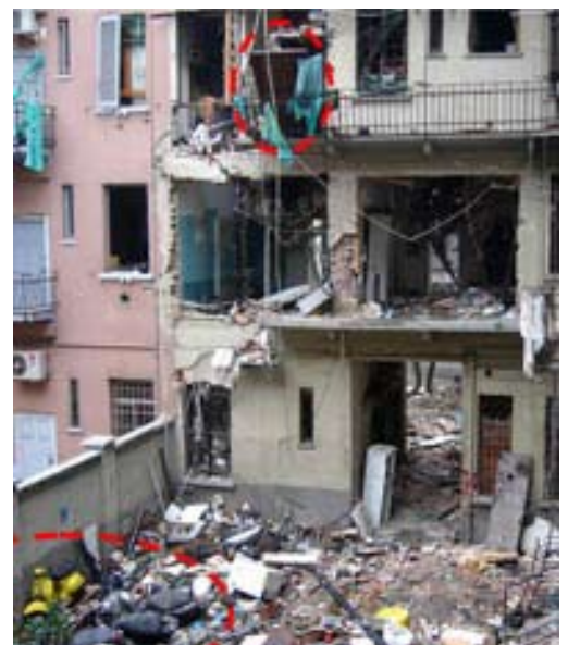
Building seen from courtyard – the shock waves from the explosion pushed the doors outwards and the moped lumped together.
