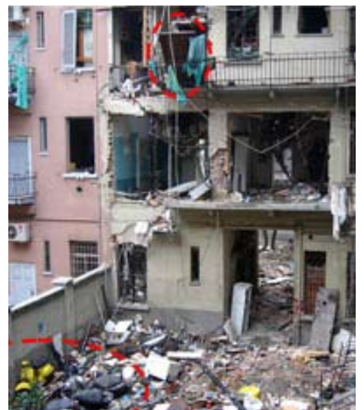
Building seen from courtyard – the shock waves from the explosion pushed the doors outwards and the moped lumped together.
